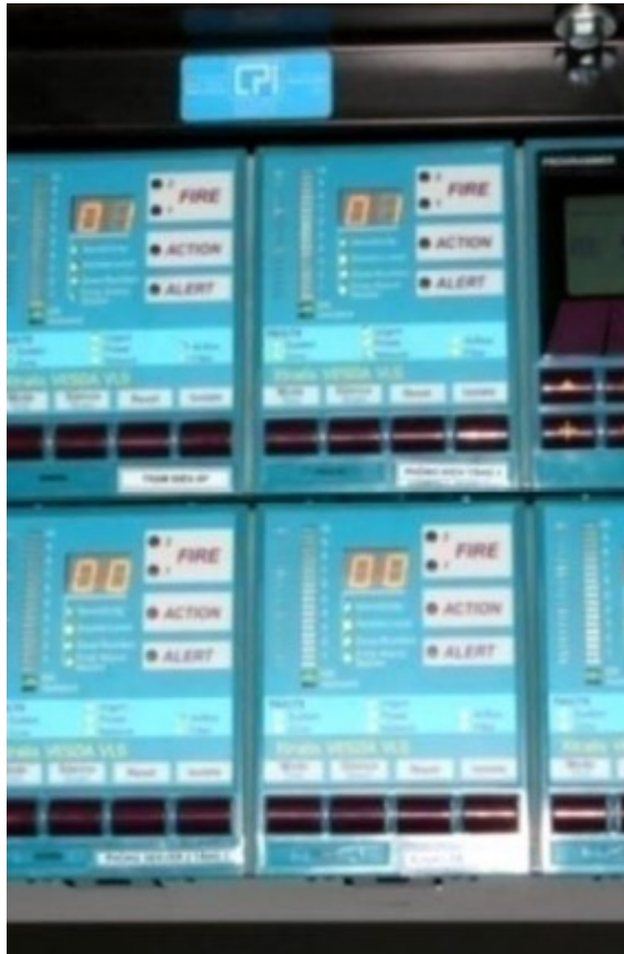
Early warning detection system (VESDA)
