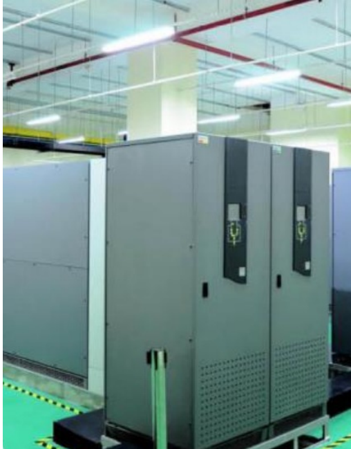
Source Transfer Switch (N+1)
